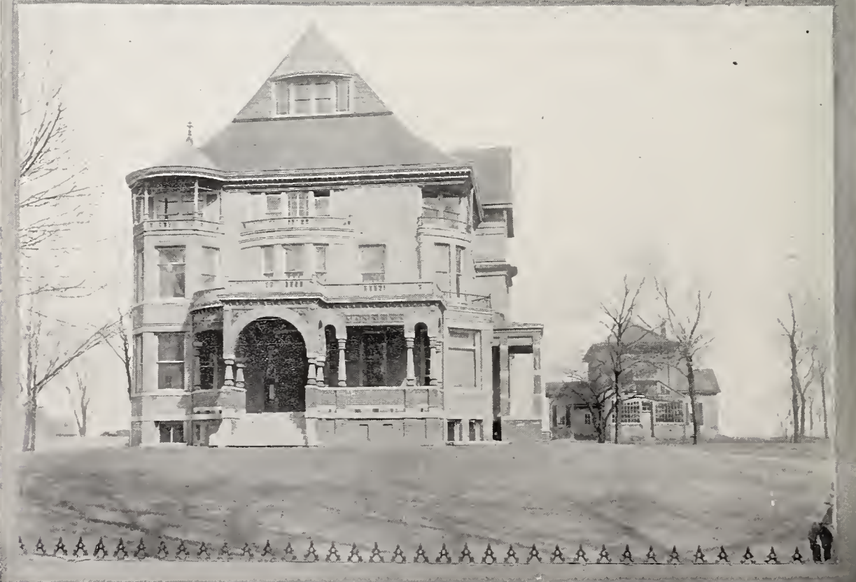
Main Building and Girls' Cottage. INSTITUTION FOR THE BLIND, JACKSONVILLE.
